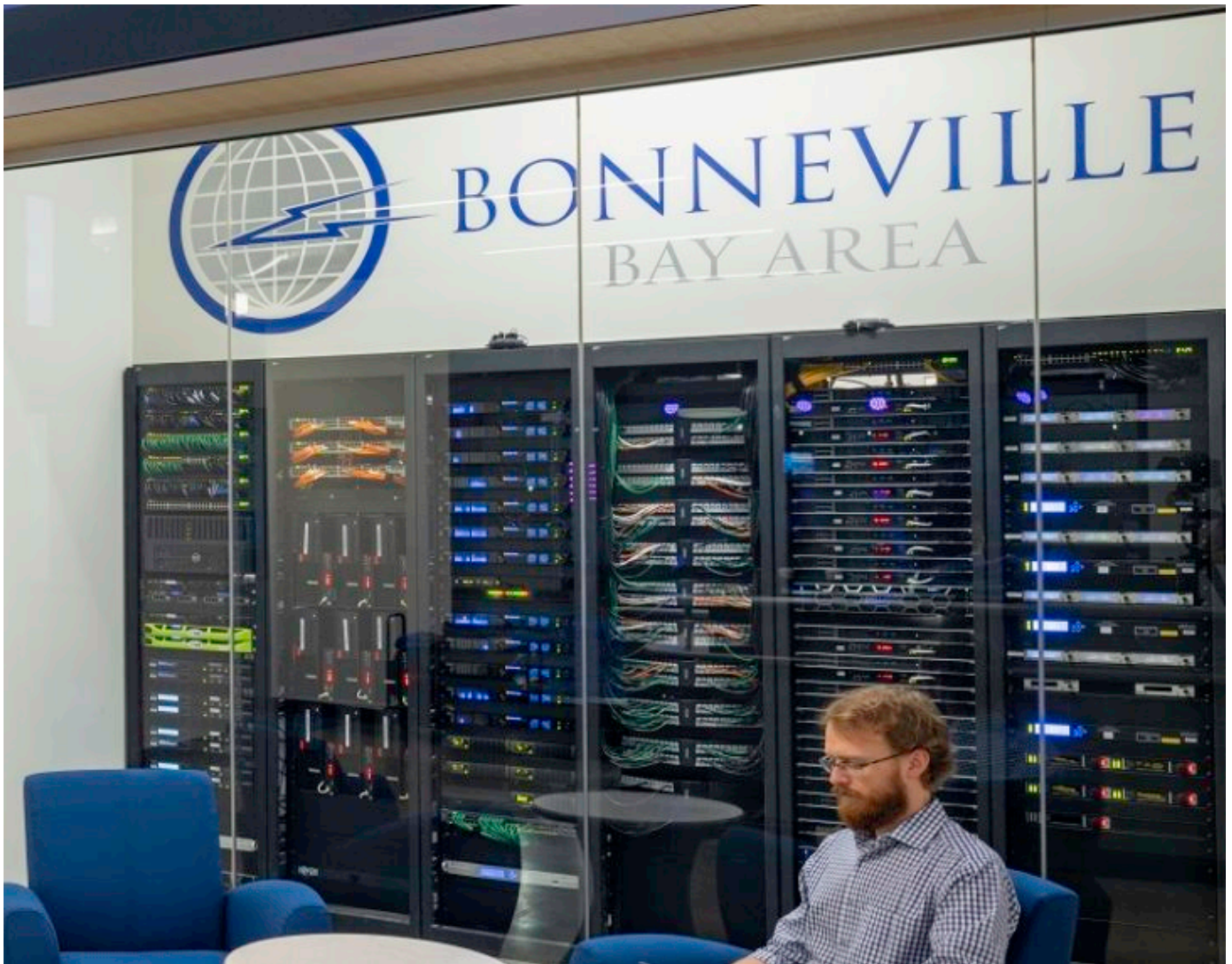
Closer view of the Technical Operations Center
